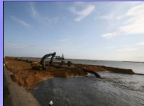
Reclamation works in full swing
