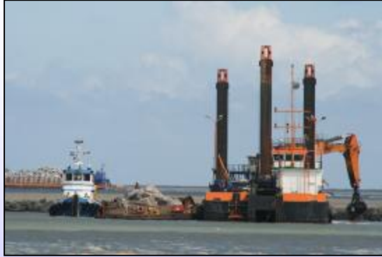
Razende Bol Installing Crest Armour on South Breakwater
