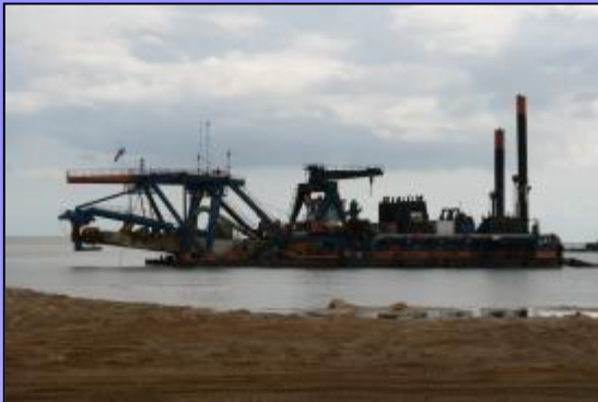
Sliedrecht 35 maintaining cutter head during dredging operations
