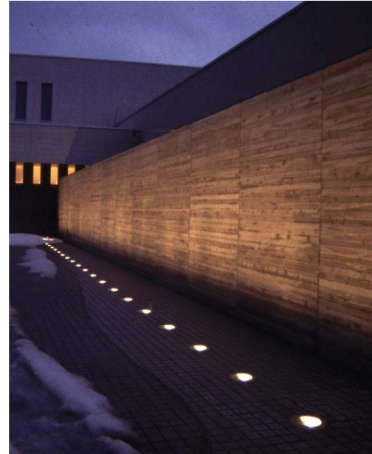
In ground uplighters providing soft wash of light revealing timber screen
